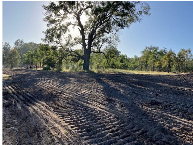
WSW sand spread at SBA3 ahead of planting
