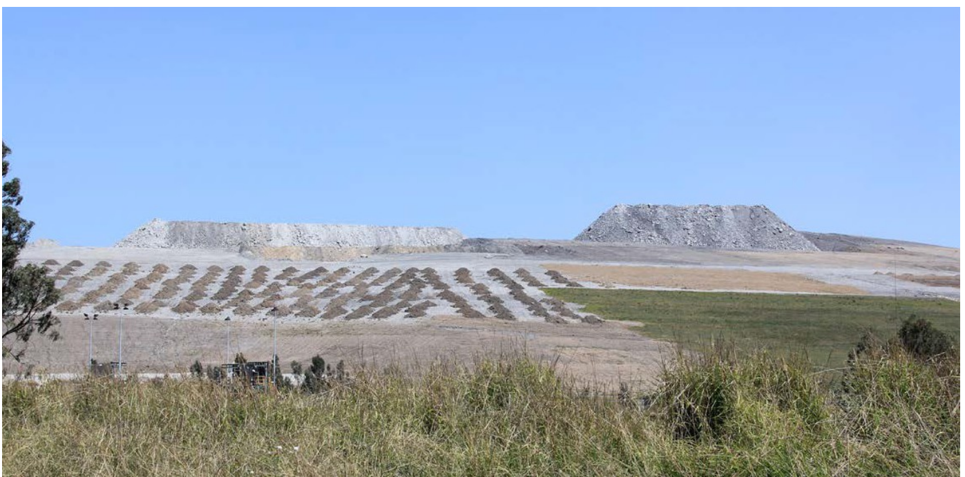
Area being bulk shaped ready for rehabilitation
